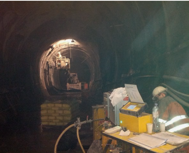
Injection and drilling work for a pressure shaft and hydropower plant
