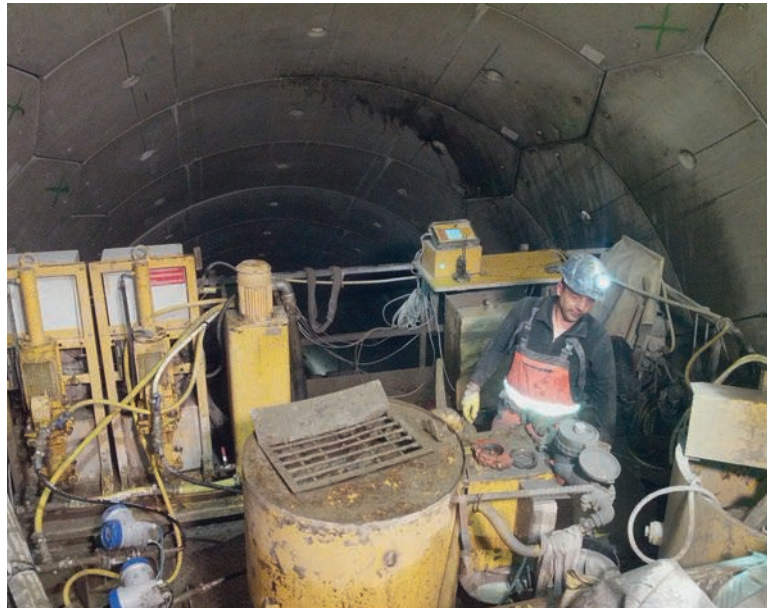
Grouting material being injected through the concrete tubings in the inclined shaft
