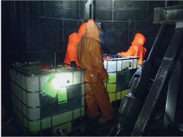
Chemical grouting material ready for the removal
