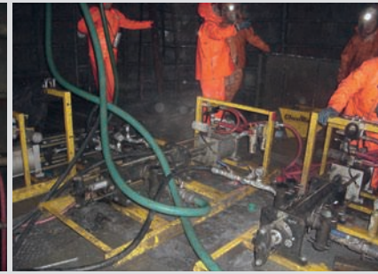
Pic. above left: Injection mounting for the sealing material "NOH20"
