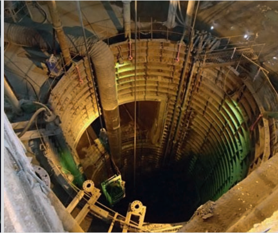
View inside the foreshaft SKS-1
