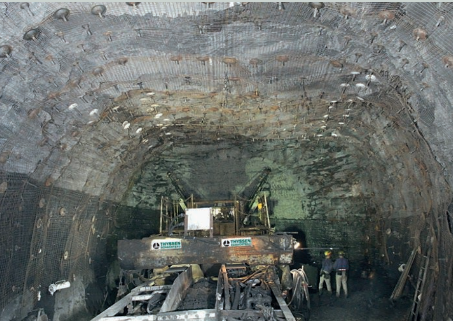
Rock bolting scheme at the roadway junction
